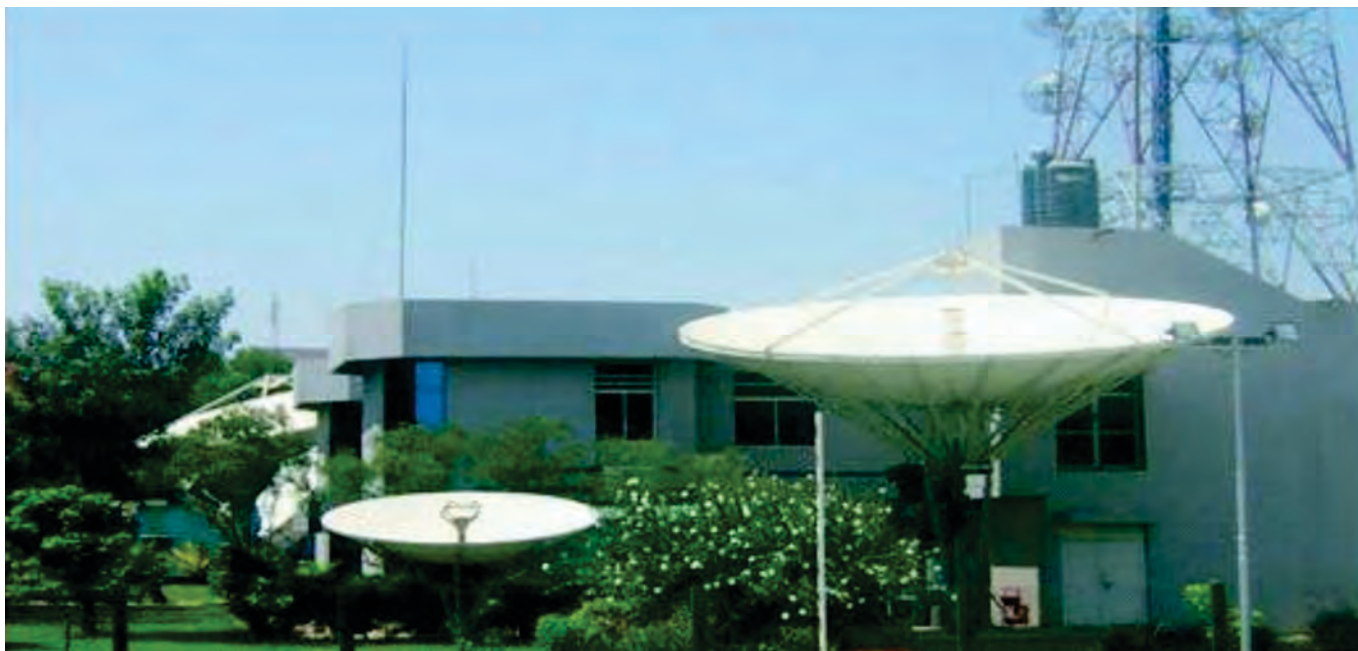
Fig. 5 : The Master earth station (MES) at ERNET India, Bengaluru
